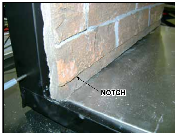
Figure 1. Notched End of Side Refractory
