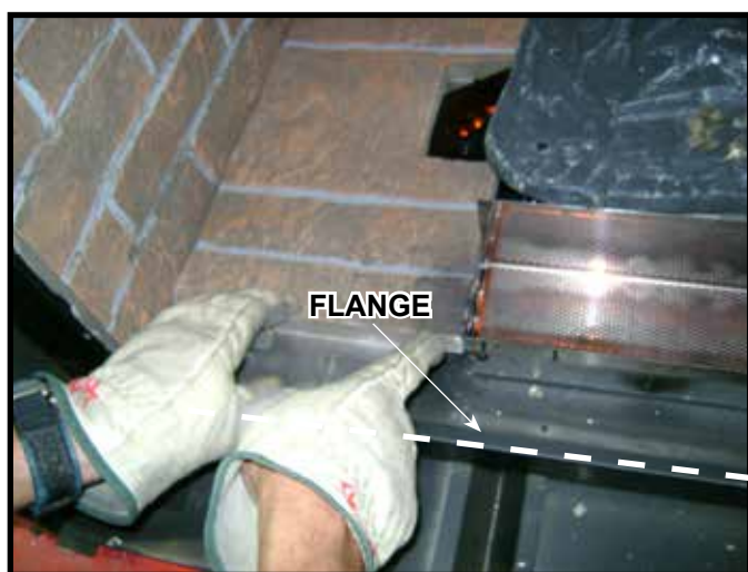
Figure 4. Positioning Left and Right Middle Base Refractory
