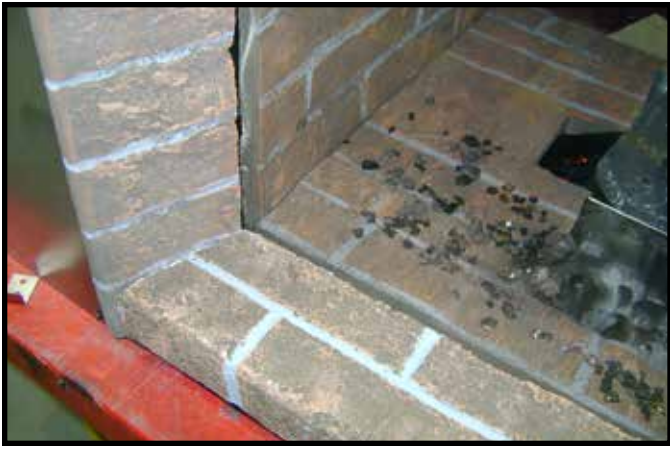
Figure 8. Outer Hearth Installation
