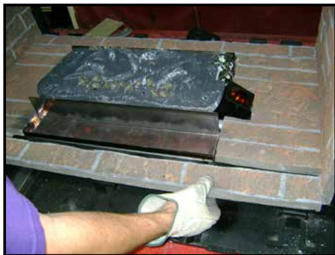
Figure 5. Positioning Outer Bottom Refractory.
